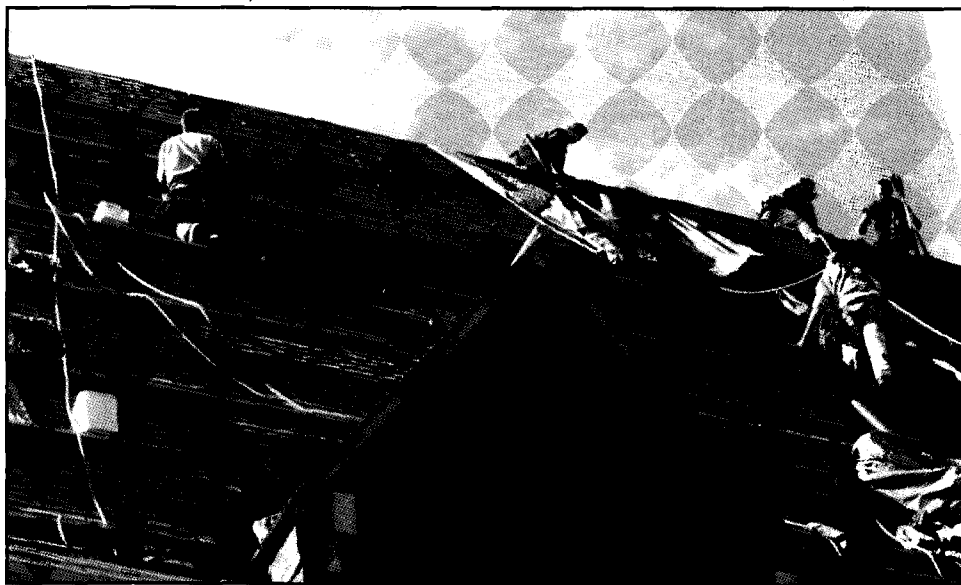
Workmen reshingling the steep roof of St. Mary's Oratory.
