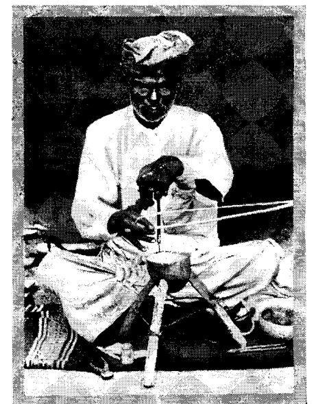
Drilling pearls in Ceylon. This is an extremely delicate operation
