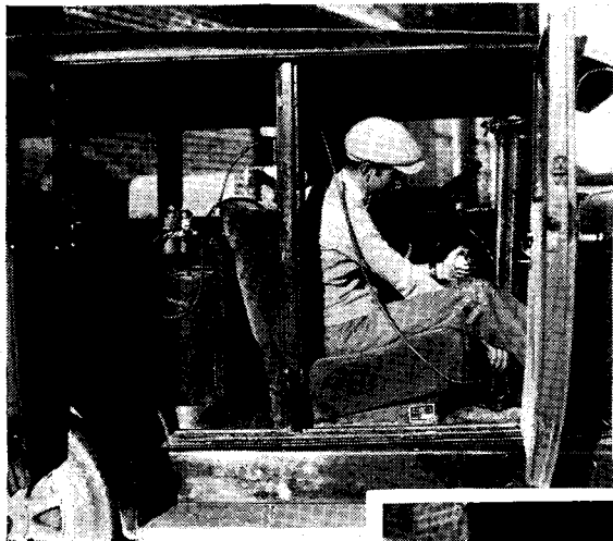
Above. The fuel consumption of a car is important to its owner. The Proving Ground device shown here measures this phase of performance—and so precisely that "miles per gallon" become virtually "drops per foot."
