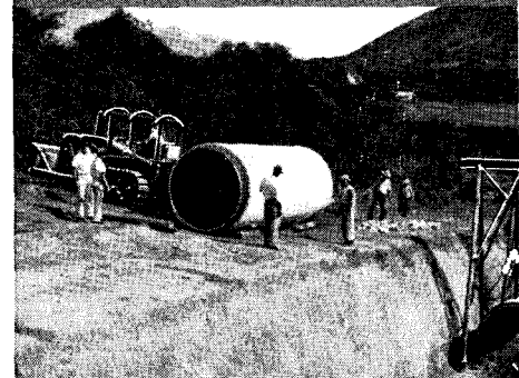
Easing 22,000-pound tubes into place. No cracks, no damage!
