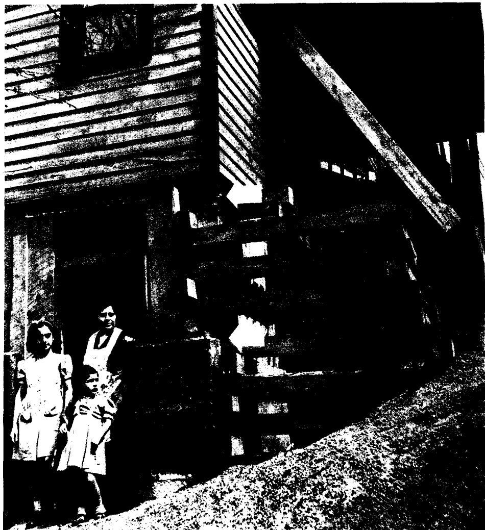
Mrs. James Lombardo and her children stand in the cellar doorway of their home. Entire rear of house and back yard settled four feet. The arrows indicate how far kitchen dropped before being shored up
