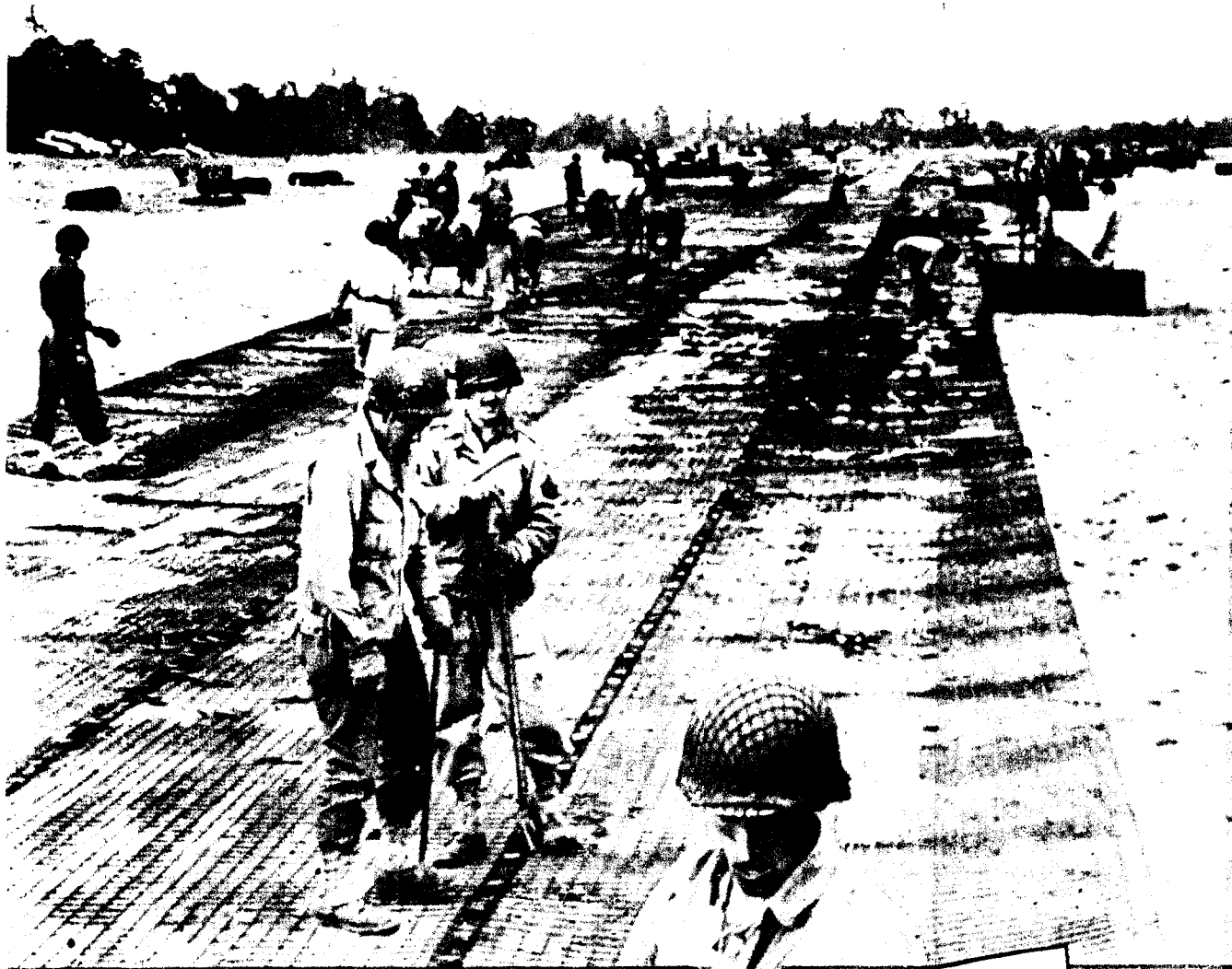
Aviation engineers, working within range of German artillery, lock together lengths of steel matting for a landing strip at a new Allied airfield
