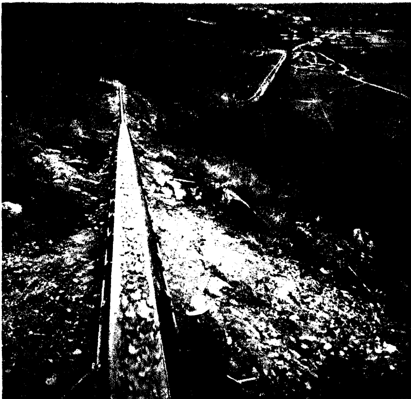
Forced to go seven miles to get rock for Bull Shoals Dam, Slocum had monster conveyor belt erected. It moved whole mountain in two years
