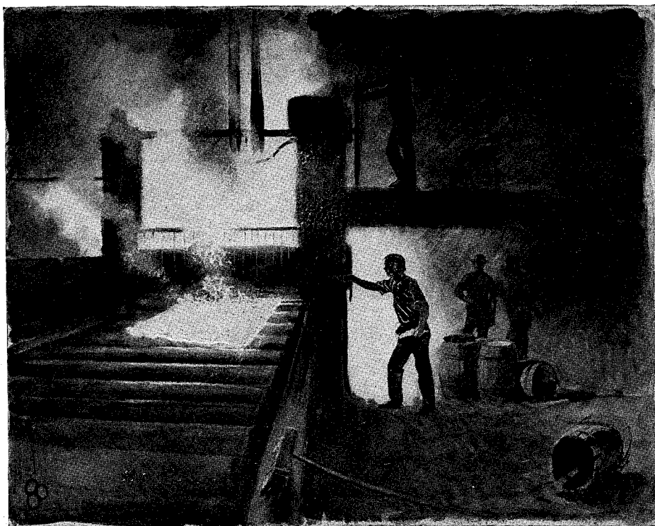
IN THE PLATE MILL: SALTING THE PLATE. AS THE PLATE PASSES THROUGH THE ROLLS THE SALT IS CRUSHED, AND THE WATER CONTAINED IN IT ESCAPES, AND, BECOMING STEAM, SWEEPS THE PLATE CLEAR OF SCALES.
