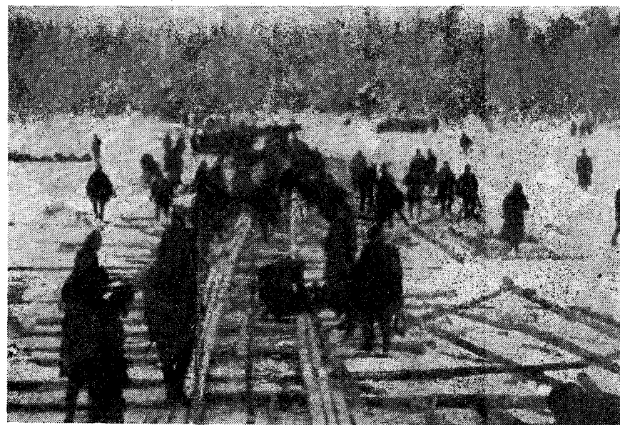
The sappers stretched a log road for the KV's.
