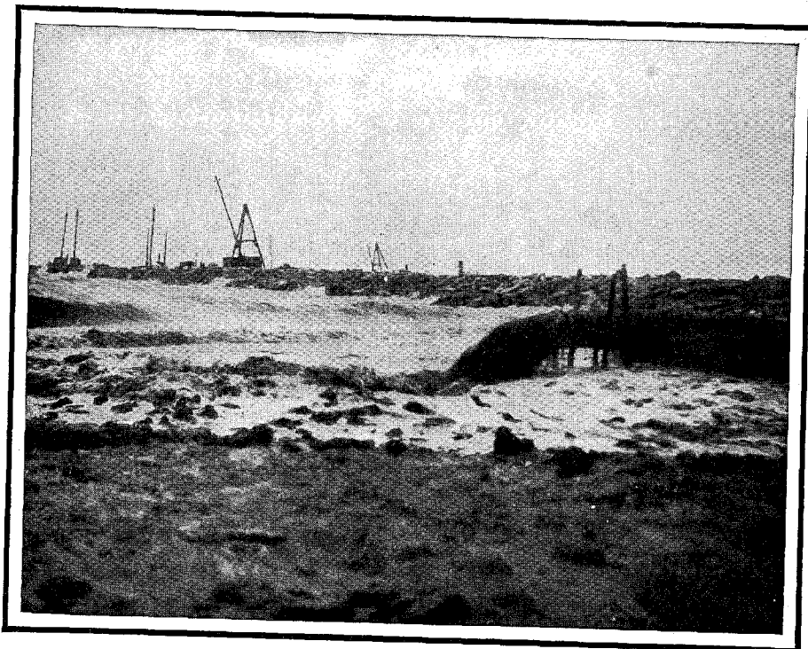
FROM THE HUGE PIPE POURS A FLOOD OF SAND AND WATER PUMPED FROM THE BOTTOM OF THE CANAL BY THE SUCTION DREDGE
