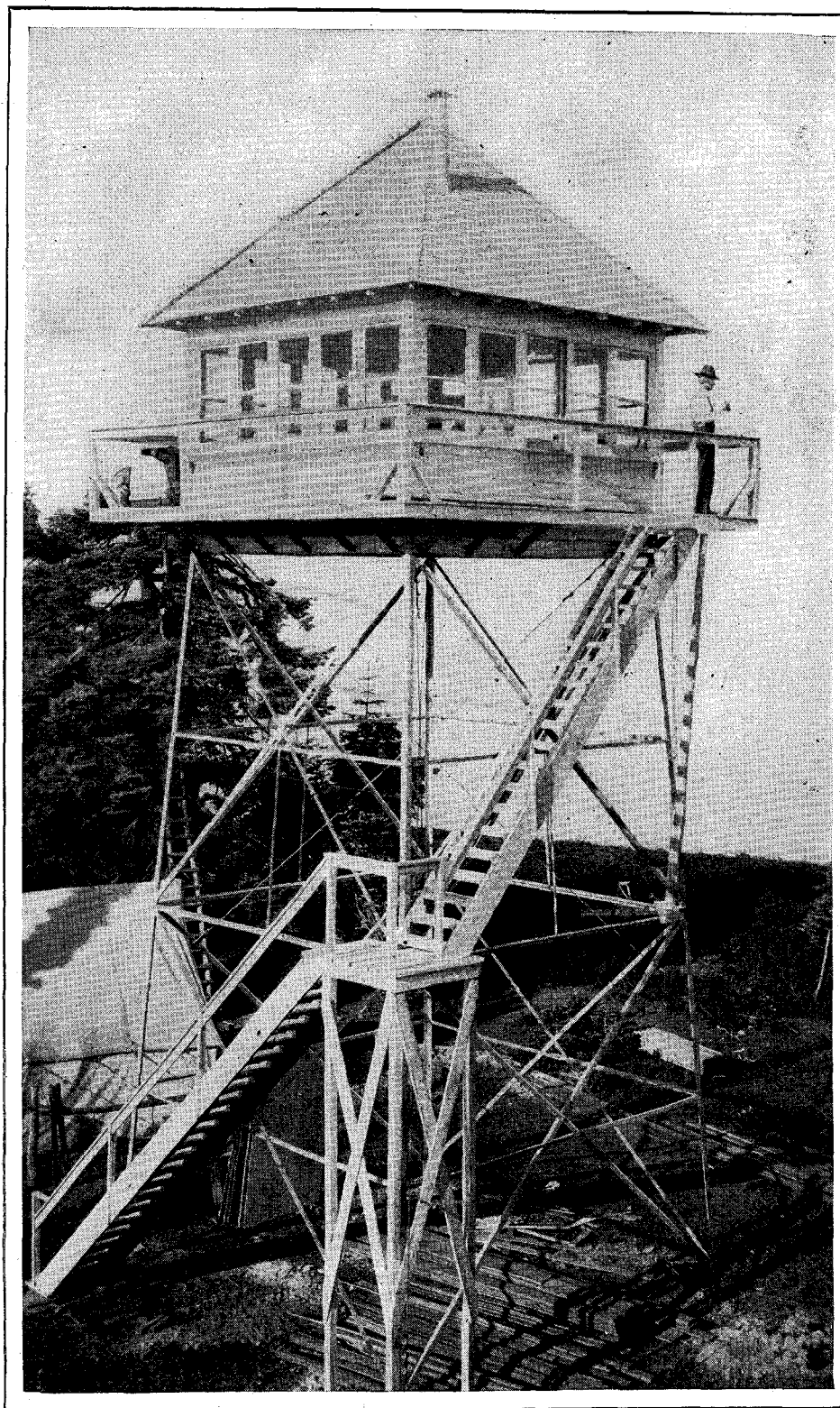
A FOREST SERVICE LOOKOUT STATION PLACED ON A THIRTY-FOOT STEEL TOWER LOCATED ON BLACK FOX MOUNTAIN, IN THE SHASTA NATIONAL FOREST
