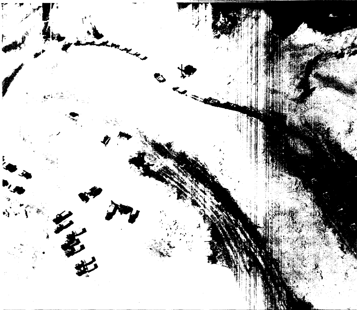
Aviation engineers ripped out four million cubic yards of coral and rock to build this B-29 base on Saipan.
